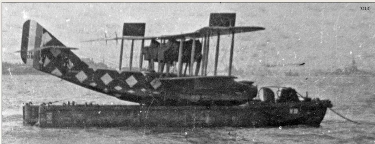
SE Saunders built Felixstowe F.2a N4083 is from the same production order as **D** and is being towed on a lighter. The lighter was another John Porte design and was essentially a mini dry dock intended to massively increase the range of the flying boats by allowing them to be towed well out to sea before taking off on patrol. Another view of this 'XXX' dazzle painted boat can be seen in the photo of N4545 on page 29.
